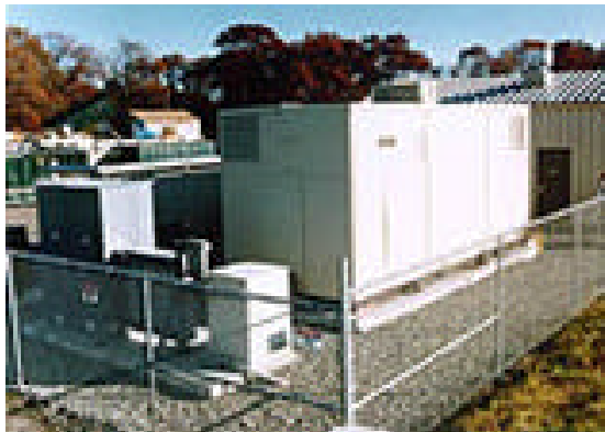
200kW PAFC power plant built by ONSI Corporation
